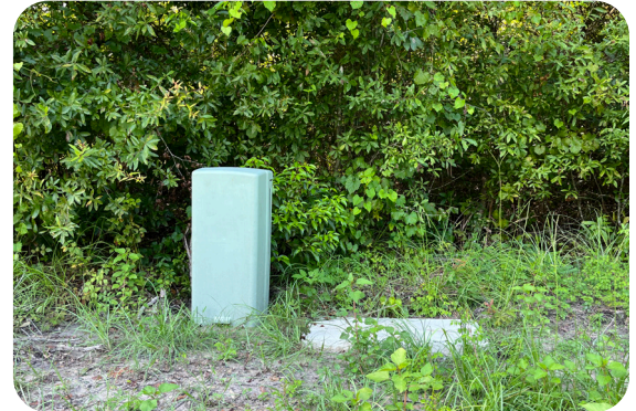
Clearfield's CraftSmart FiberFirst Pedestal sits next to a small slack storage vault.
