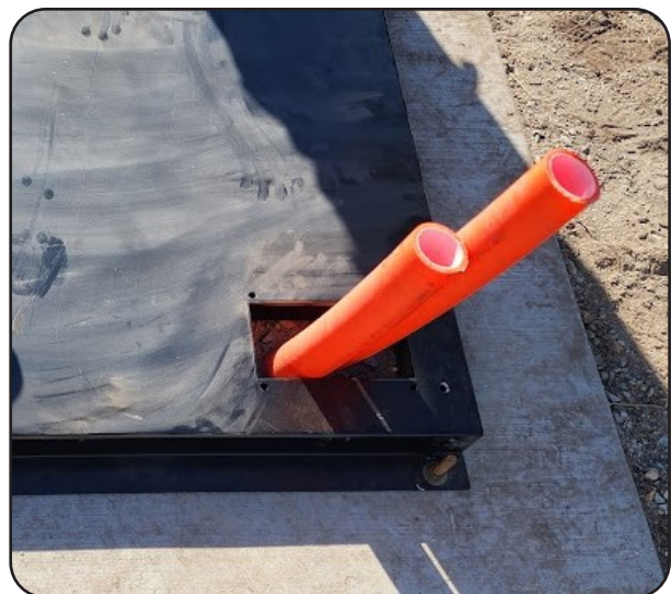
Seal conduit area with sealing foam provided
